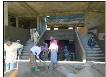
Construction on the Axumite Heritage Foundation Library in Axum, Ethiopia.
